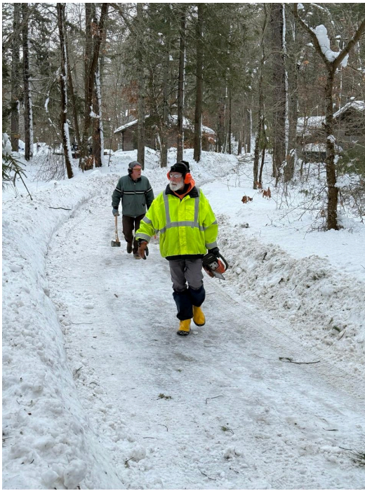
Ted and Dennis heading to clear trees limbs from the downed power lines.
